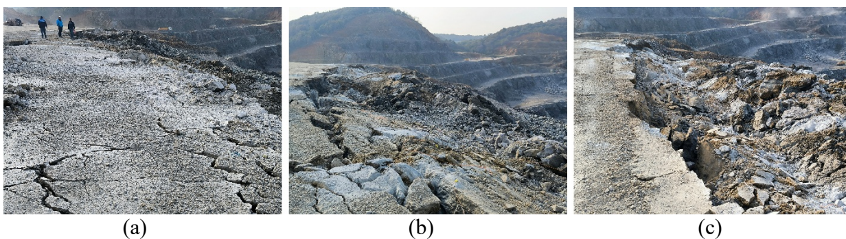
Figure 3. Back-break network observed in (a) Zone I, (b) Zone II, and (c) Zone III of the first blasting operation
